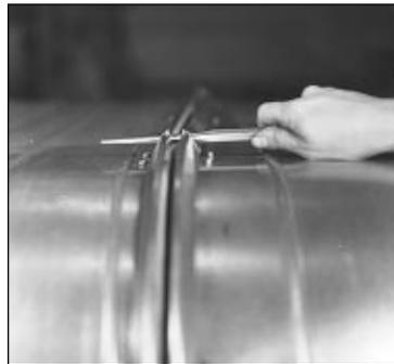
17. Align mating frames. A drift pin can be used to correct any misalignment. Compress gasket with clamps.
