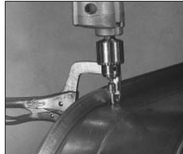
10. Work in one direction around duct when seating the frame. Fasten in sequence as you go.
