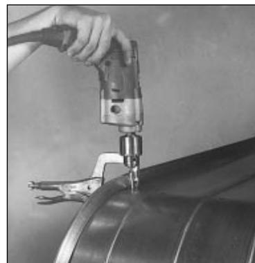
12. Continue in one direction around the duct at evenly spaced intervals as per the schedule below. Place last fastener within 1" of the end of a straight or curved flange section.
