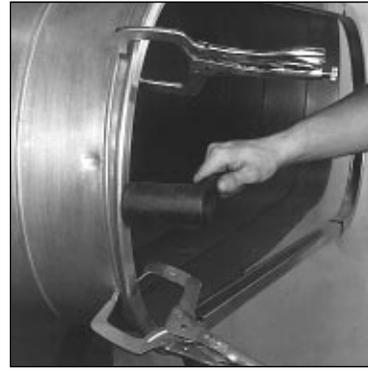
8. Use a mallet to seat the Ovalmate frame onto the duct. Do not hammer the center of the major axis. An inward curve could occur. Make sure cut edge of the duct is square. Metal to metal contact is preferred between duct and frame but you may have to adjust in order to square the connection.
