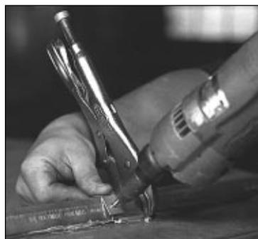
20. Now press the cleat into position and fasten with a metal screw. Install at intervals according to the following schedule:
