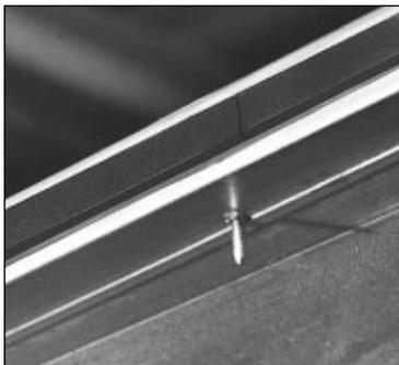
16. Apply Neoprene Gasket completely around Ovalmate frame to the beginning point. Where gasket meets cut so ends butt up against each other.
