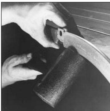
7. If the raw edge of the duct gets caught behind the Ovalmate connector piece, press the duct with your fingers while tapping the frame in order to assure that the duct will be correctly seated into the integral mastic.
