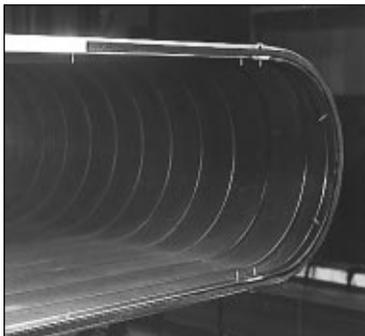
14. Start applying Ductmate Neoprene Gasket Tape to the face of the straight Ovalmate angle about halfway between connector pieces. Position gasket in the center of the Ovalmate angle as in photo. When crossing connector pieces place the gasket over the raw edge of the duct.
