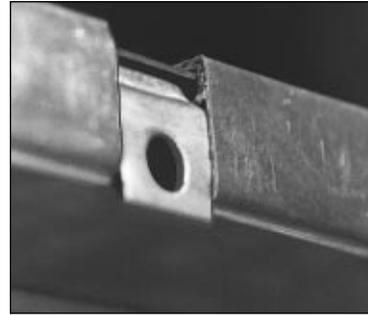
9. The duct must be seated all the way into the Ovalmate angle in order to penetrate the integral sealant and avoid air leaks. Double check to make sure that the duct edge protrudes past the downset of each Ovalmate connector piece.
