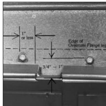
11. Begin securing the leg of the Ovalmate flange to the duct section by clamping seated frame close to one of the Ovalmate connector pieces. Place a pop rivet, screw or spot weld within 1" of the flange end and no closer than 3/4" or further away than 1" from the face of the flange.
