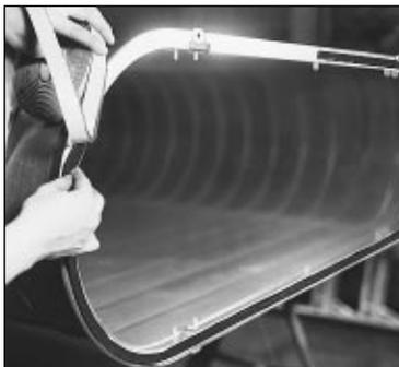
15. Press gasket firmly into contact with the face of the Ovalmate flange and the connector pieces. Ductmate Neoprene is the preferred gasket.
