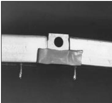
13. On all Ovalmate connector pieces apply Ductmate 440 Gasket as in photo (approx. 3"). Position 440 Gasket so that it covers the raw edge of the duct protruding past the Ovalmate connector pieces.
